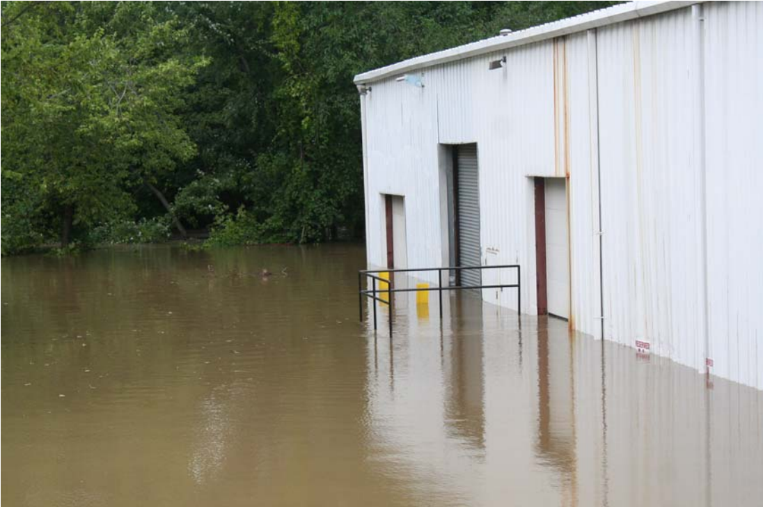
Saw Mill River Road, Ardsley, New York
